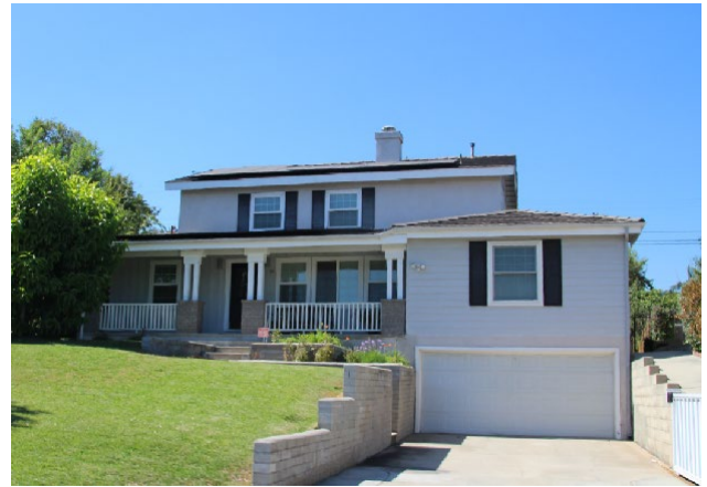
Split-level design reduces need for intensive grading of a site, maintaining natural terrain
